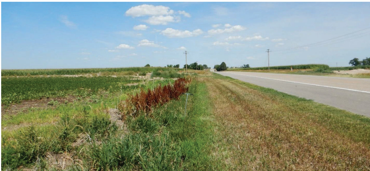
Typical view along US-26 and L62A showing rural 2-lane highway, shoulder, roadside ditches, and farmland.
